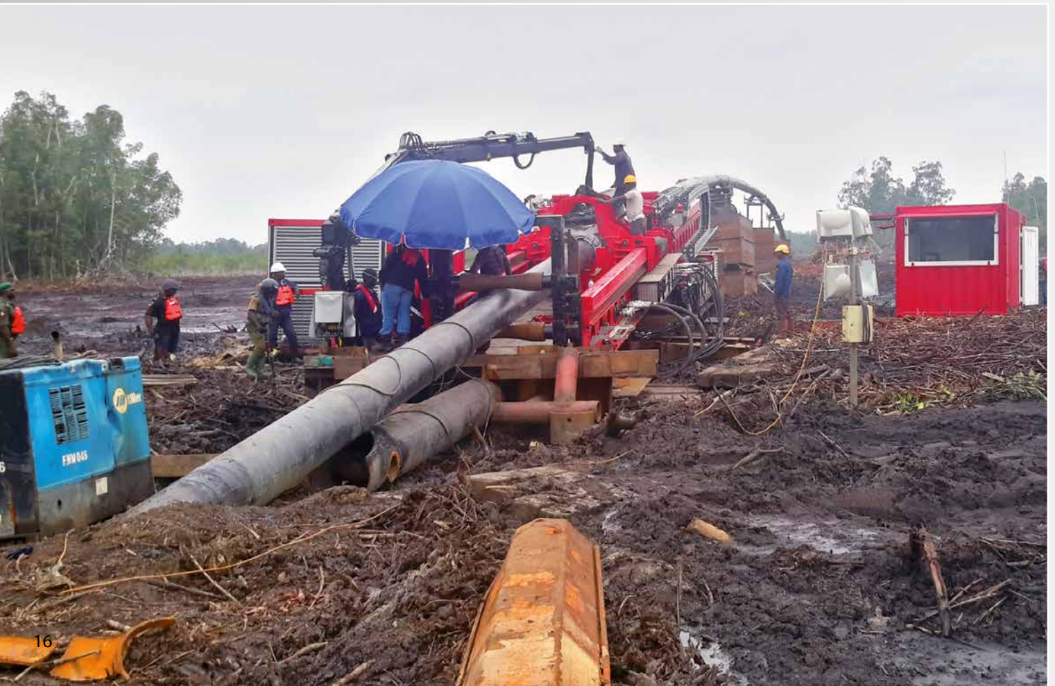
HDD-rig with integrated Pipe Pusher
