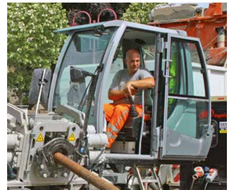
90° rotational control cabin including heating and air conditioning
